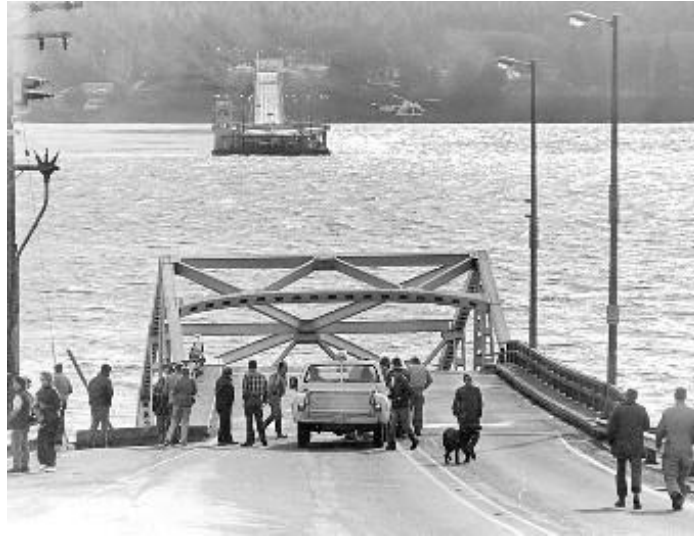
Hood Canal Bridge shortly after collapse 1979
